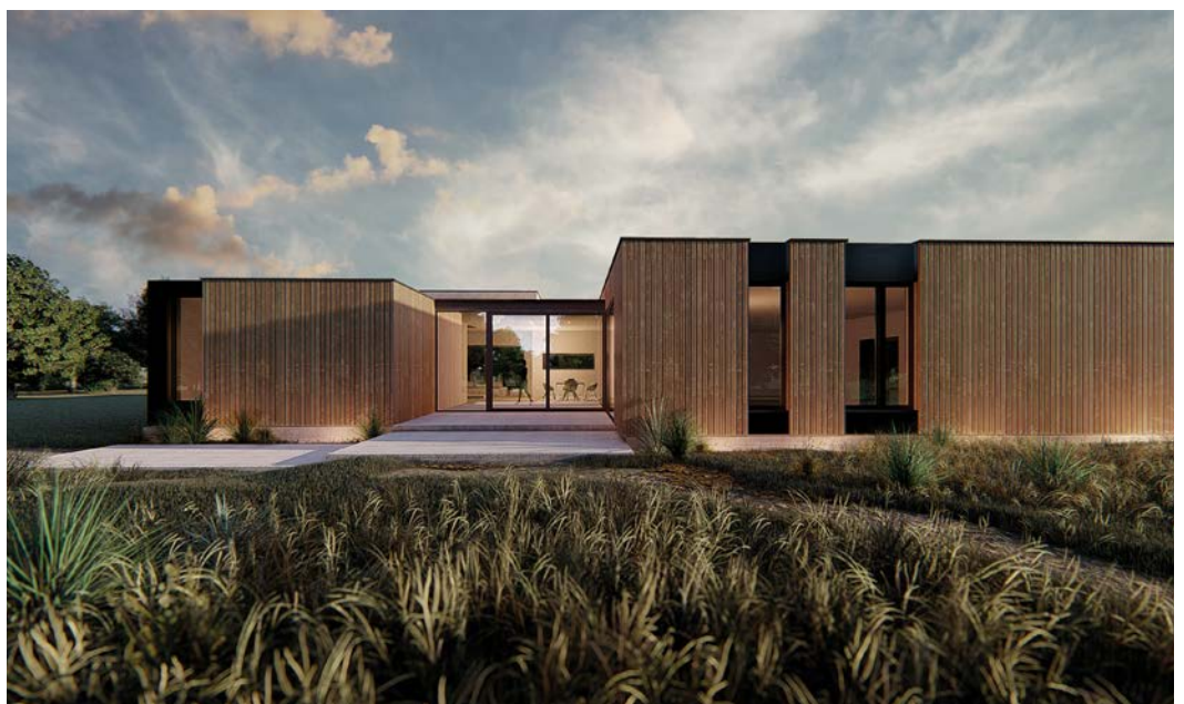
UTV channel profile ThermoPine façade.
